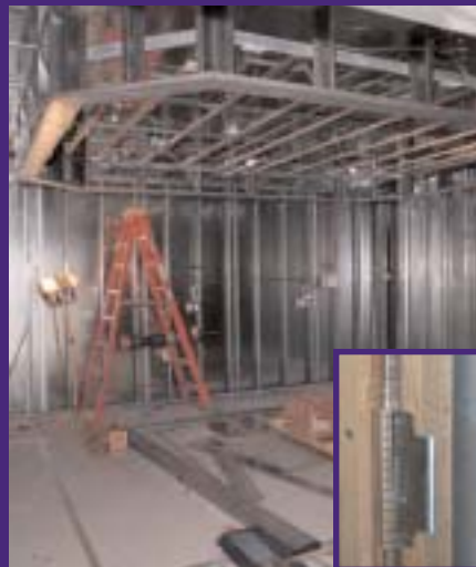
Right: Copper shielded walls, doors and windows have been installed to isolate the magnetic resonance imaging from radio frequency interference.
