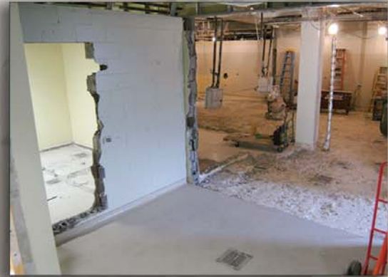
Modifications are made to the area where the ICU's central work station and adjacent isolation room will be located.
