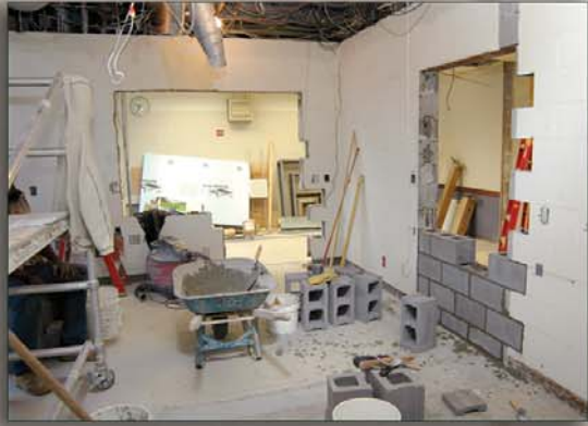
With the office area enlarged, new windows under construction in the emergency/discharge area.
