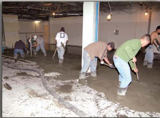
Concrete is poured for the new floor in the ICU.
