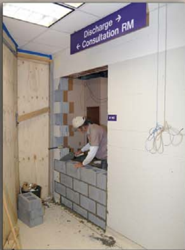
Cinder blocks go up for the discharge window.
