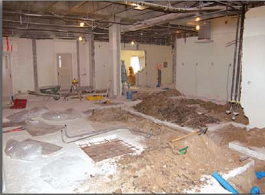
Walls have been torn down, floors removed and new plumbing is being installed in the future ICU.
